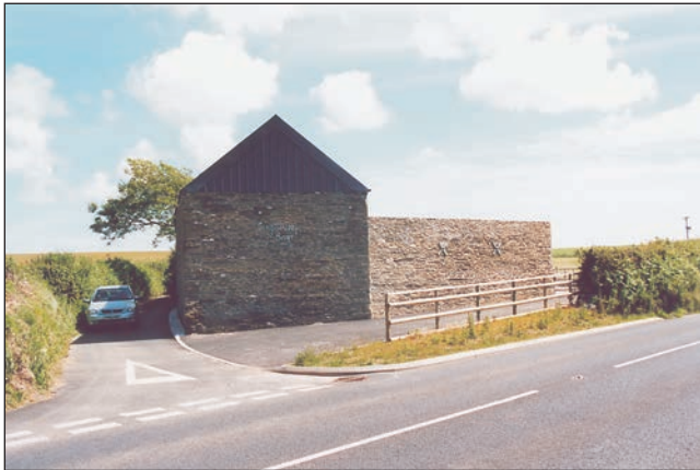
Above: The wind-shaped tree behind this isolated field barn suggests the high stone wall at right was built to shelter its yard from the weather. With a view to retaining its value as a visual barrier too, the wall's repair went hand-in-hand with the introduction of a new business use.
