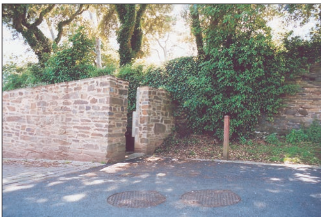
Below: Integrated with existing stone walls and built of locally salvaged materials, these new stone walls serve to disguise a refuse collection point near the entrance to a courtyard group of converted farm buildings.
